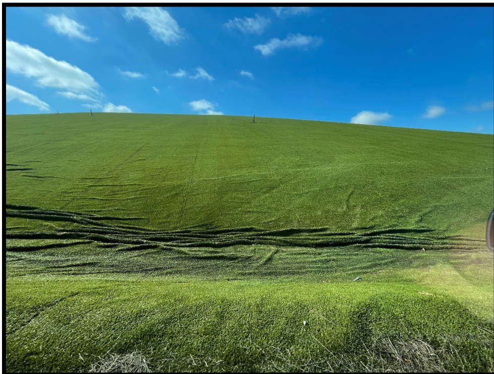
Photograph 4: View of rills in closure turf on the north side of Area 1-2.
