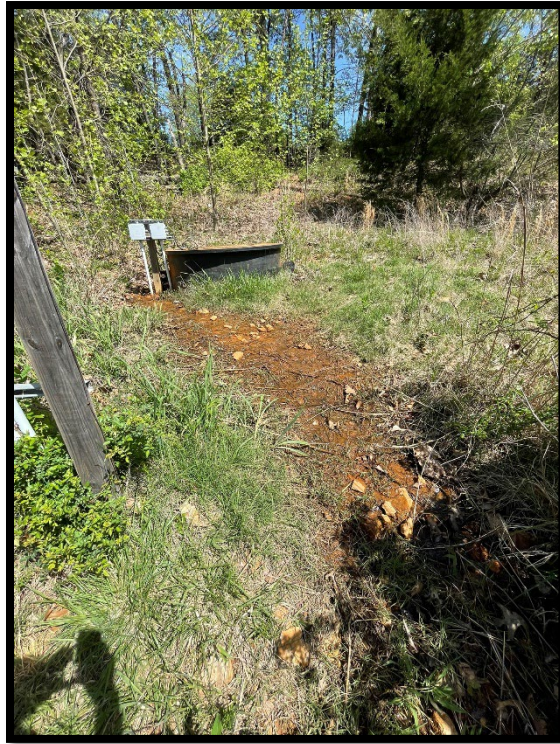
Photograph 1: View of erosional rill from VLCS-1 overflow.
