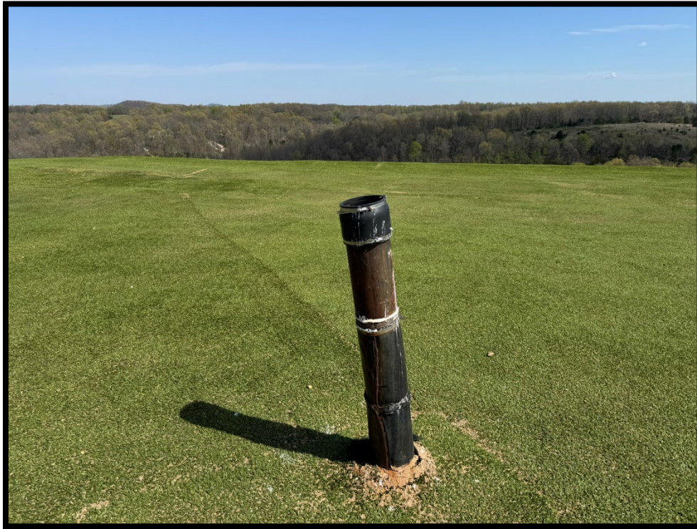
Photograph 5: View of detached turbine vent on north side of Area 1-2.
